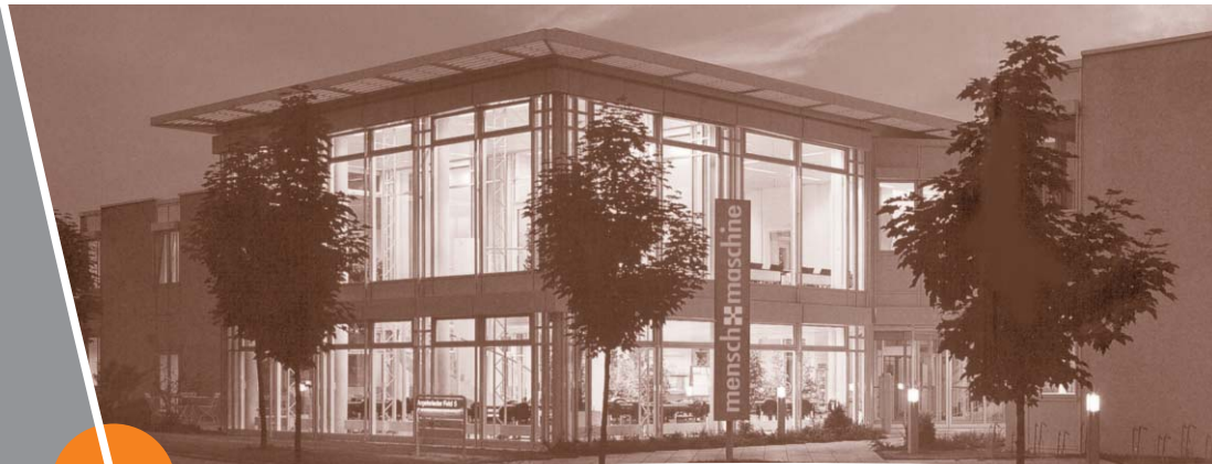
The M+M headquarters building in Wessling near Munich
