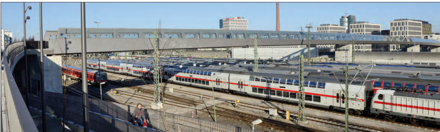
Photocredits: Hans Gössing (1/2), SSF Ingenieure (3/4/5)
